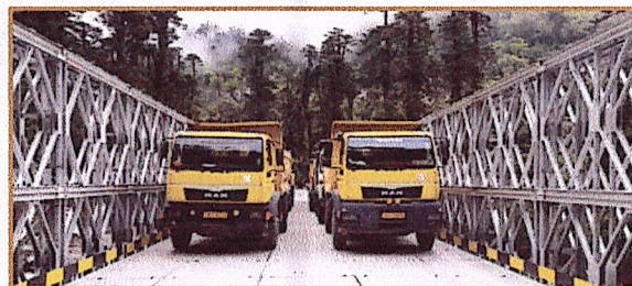
GRSE Built 140 Ft Double Lane Modular Steel Bridge at Flaghill, Sikkim
